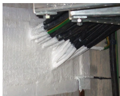
Electrical Shaft Sealing
