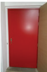
Fire Rated Electrical Shaft Door
