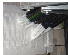
Electrical Shaft Sealing
